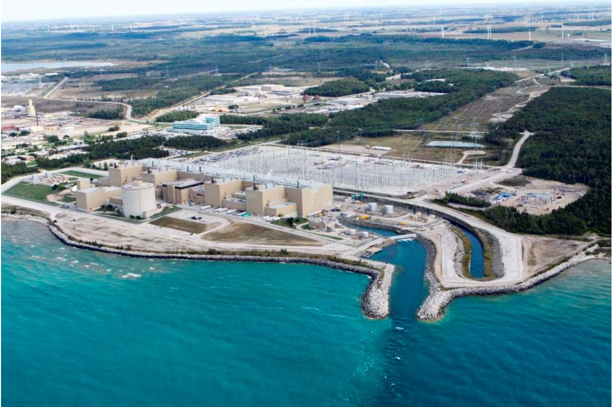
Figure 8: Aerial Image of Bruce B Station at Bruce Power
